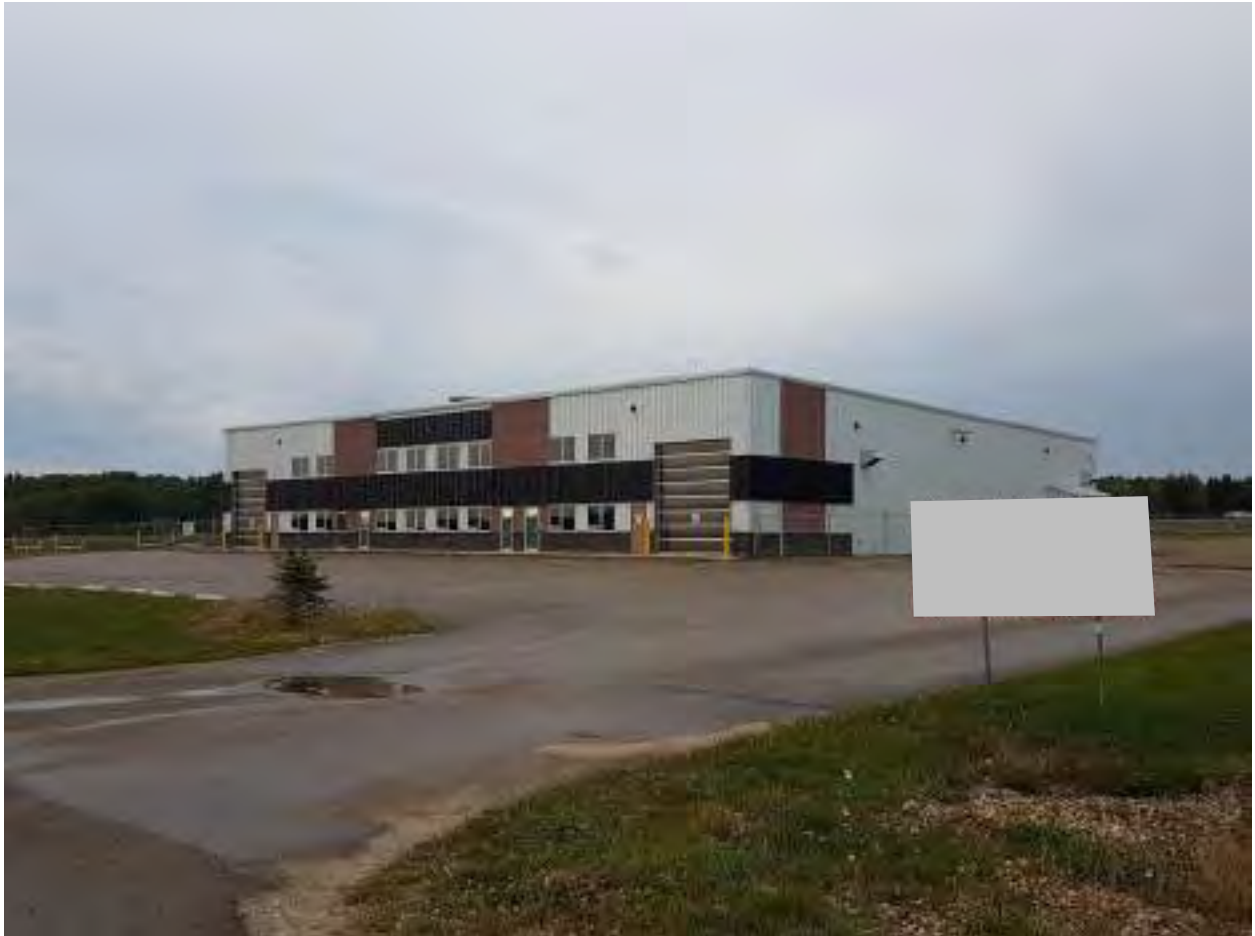
North Facing From 58 Avenue
