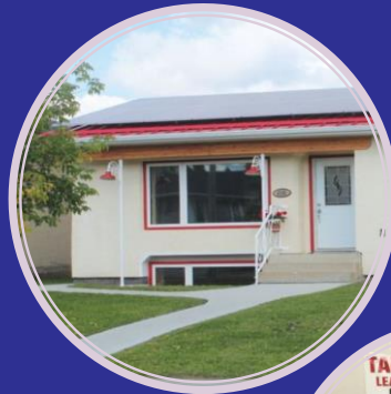
Straw-insulated, solar PV powered residential home
