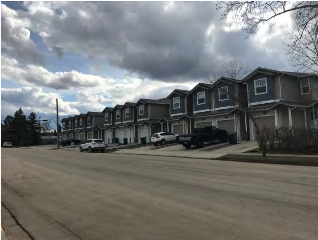
The nearby row housing to the south of the parcel from 46 Street
